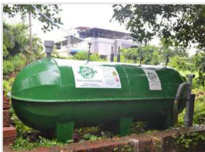
Figure 11: Examples of containerized composting (left-up, left-down, and middle-down), small-scale material recovery and transfer station (right-up), 1 and small-scale bio-digester (right-down) 2
